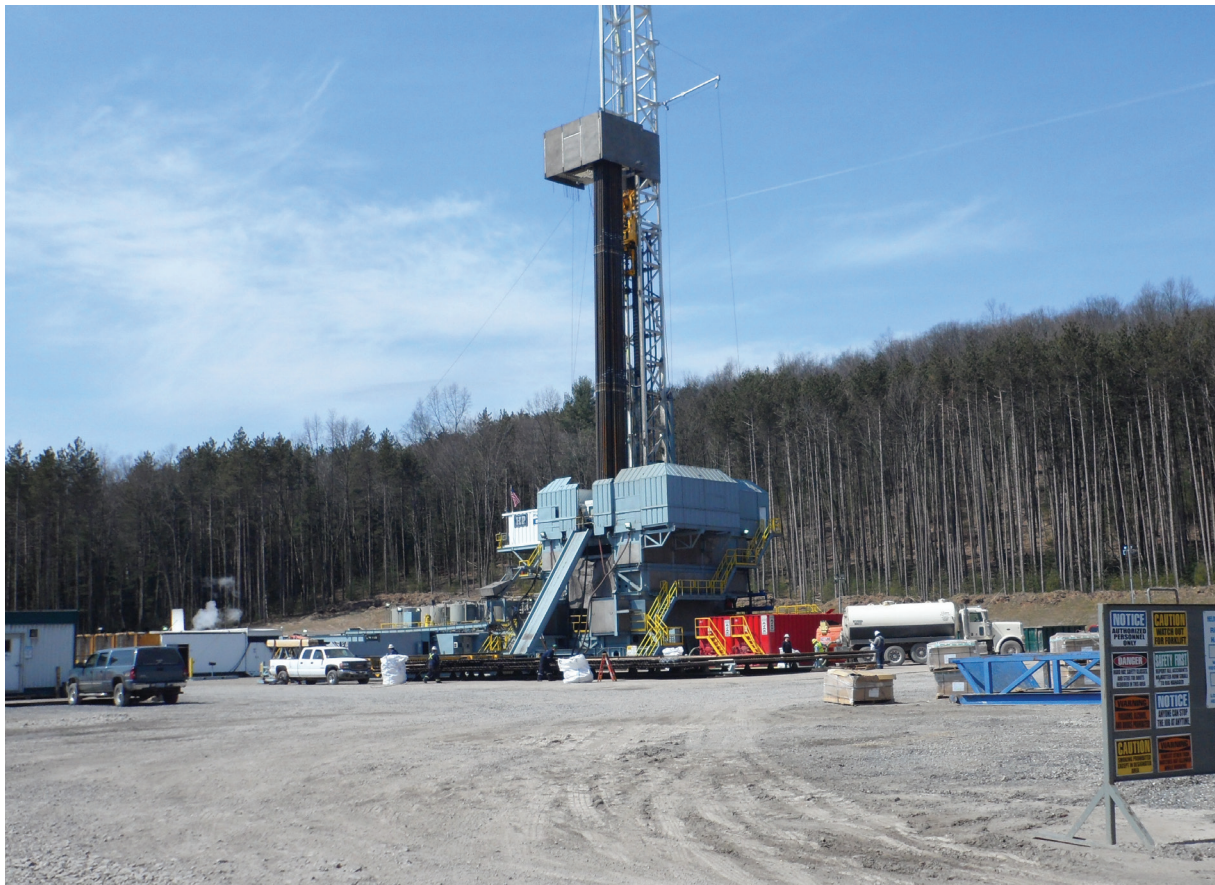
A Marcellus Shale drilling site in Pennsylvania © Penn State
